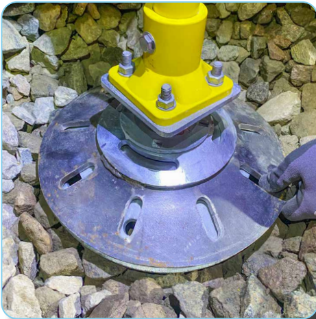
Above: Anchor Screw being driven into ground with torque head and power pack. Right: Interface plate being aligned to installed Anchor Screw. Line of installed Anchor Screws in the ground.
